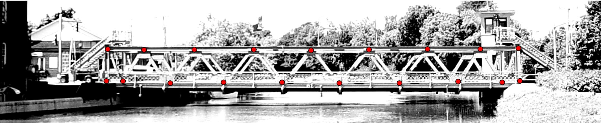
Each side of the main street bridge in Brockport, NY has 19 joints, 35 members, and three reaction forces (pin and roller), making it a statically determinate truss.
